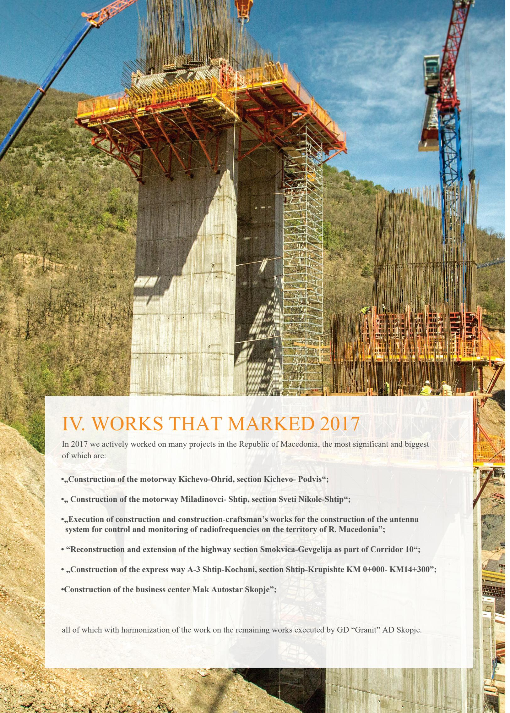
A large-scale construction site for a bridge or highway infrastructure. The image shows two tall, cylindrical concrete pillars under construction. The pillars are surrounded by extensive scaffolding and rebar structures. Two large cranes, one blue and one red, are positioned around the site. The background features a hilly landscape with sparse vegetation under a clear blue sky. The text is overlaid on a semi-transparent white box at the bottom of the image.
